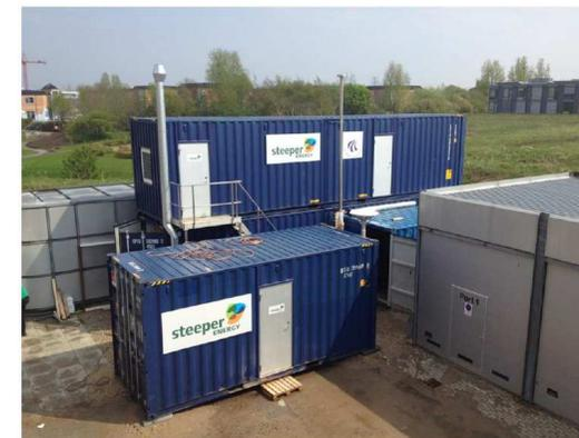
Figure 10: CBS #1 set-up at Aalborg University Campus, Denmark. Container in the front contains the pretreatment unit, the 2 containers in the back contain the process plant in the bottom and the control and utility system in the top.
